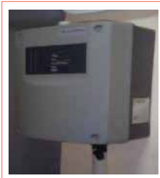
Earth Rite Relay System automation for solvent unloading
