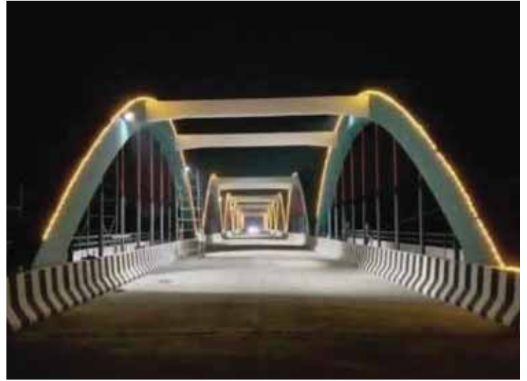
Coating application on Korapuzha Bridge, Calicut, Kerala
