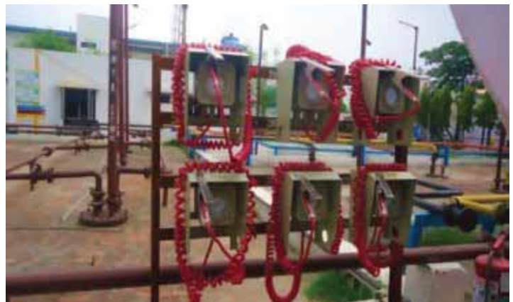
Earth Rite Relay System automation for solvent unloading
