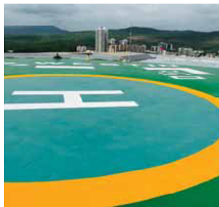
Leading Hotel Helipad work completed with Luxurea MP 500 and Pro Polyshield UV 75.
