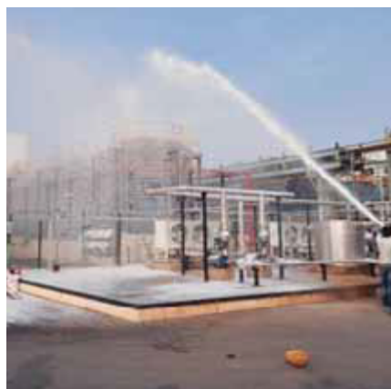
Foam Bladder Tank assembly and foam monitor in operation
