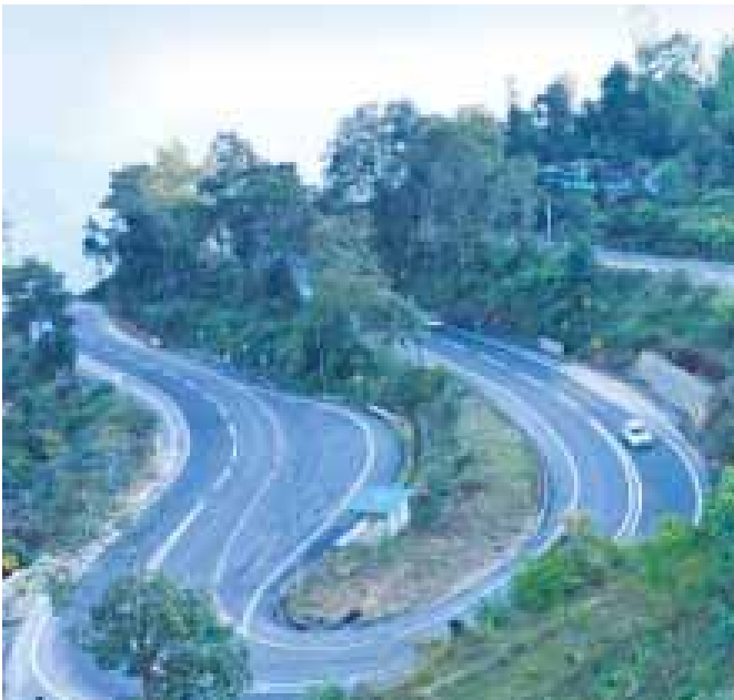
Thermoplastic Road Marking (Sigmark) at Rehnok-Pakyong Road Project- Sikkim (National Highway- 717A)
