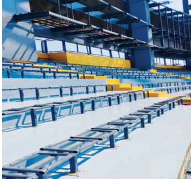
Renowned Stadium Rehabilitation work completed in record 60 days, of stands and structures, with Pro Polyshield UV 75 and BR PU High Gloss Enamel.
