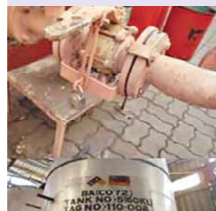
Color coded unloading valve with lock and key and Tank with same color
