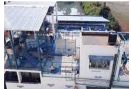
Modern and compact ETP set-up at Naltali Plant
