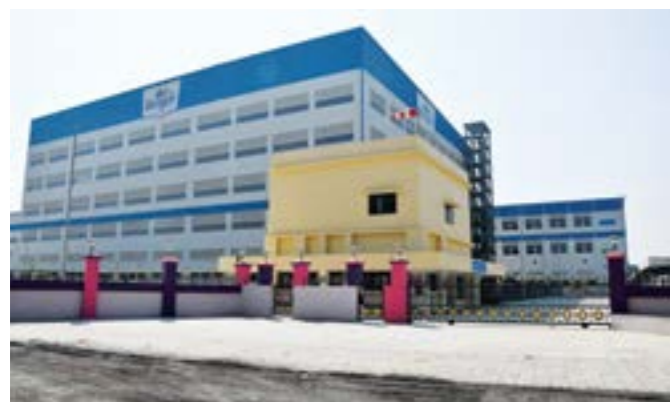
New Sandila (Uttar Pradesh) plant
