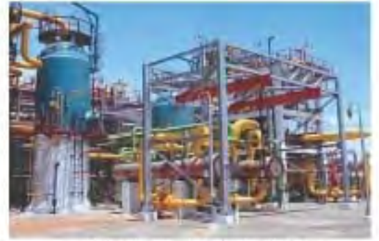
Petrochemical Project with high performance Protective Coatings
