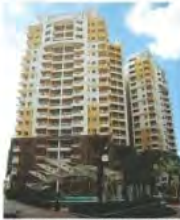
Project - Mantri Greens, Bengaluru
