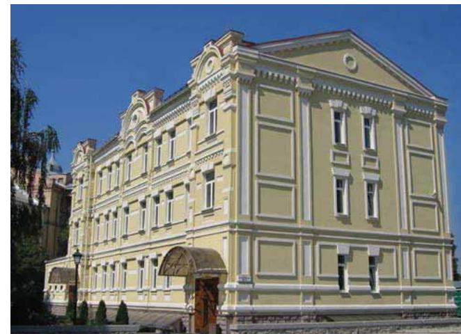
Office building in Kiev, Konstantinowska Street, 32B. ETICS with EPS Board. Year of completion 2005
