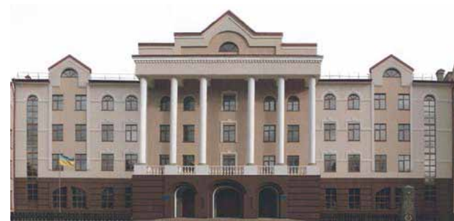
Nizhyn Agrarian University, Nizhyn, Ukraine. ETICS with EPS Board. Mosaic render. Year of completion 2015-16
