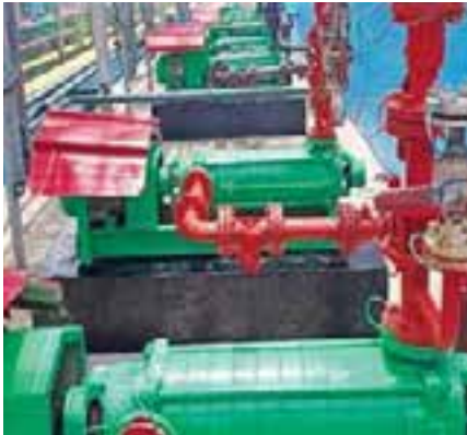
Conventional Pump seals are replaced with Mechanical seals which ensures no leakage and spillage free dykes.
