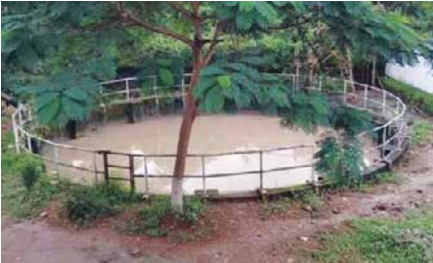
Rain Water Harvesting Pond at Goa Plant Total Storage Capacity - 540 KL
