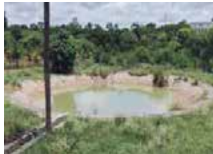
Rain Water Harvesting Pond at Hindupur Plant. Total Storage Capacity - 600 KL
